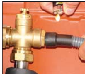
Protection hose to shrink on the flow line connection (hot air ...)
