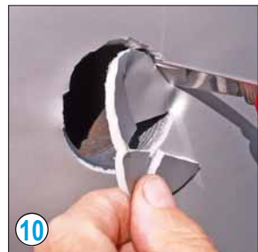
10 Carefully cut out the holes
