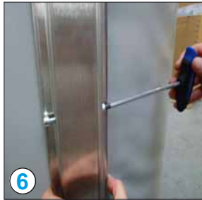
6 Fasten all hexagon socket screws and check if the insulation jacket fits tightly.
