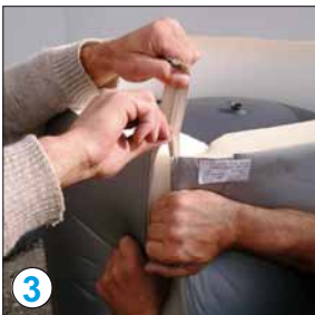
Watch out when closing the zipper (danger of tearing the insulation when not warm enough) Do not use a tong or any other tool.
