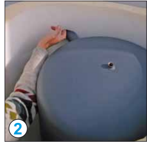
Adjust sockets to insulation
