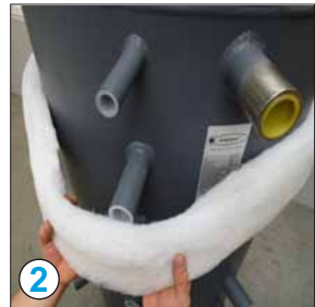
2 Pull the insulation ring for the tank's pedestal from top ...
