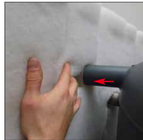
3 Put insulation around the tank and pass the sockets through the pre-cut holes (do not remove the foam plugs from the pre-cut holes that won't be used)
