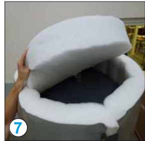
7 Put insulation on top of the tank (pay attention to the position of the sockets)
