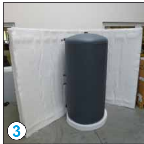
3 Put insulation around the tank and pass the sockets through the pre-cut holes (do not remove the foam plugs from the pre-cut holes that won't be used)
