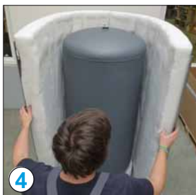
4 Tightly enclose the tank with the insulation
