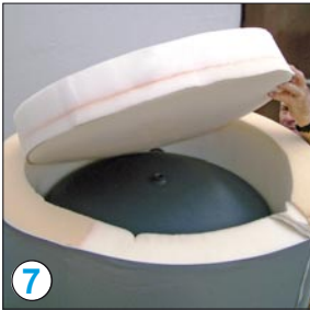
Put on the insulation cap and its cover
