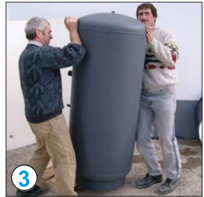
Lift the tank of the pallet
